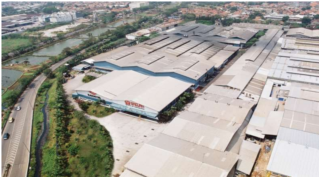
Kapuk Plant (Radiator Facilities)
